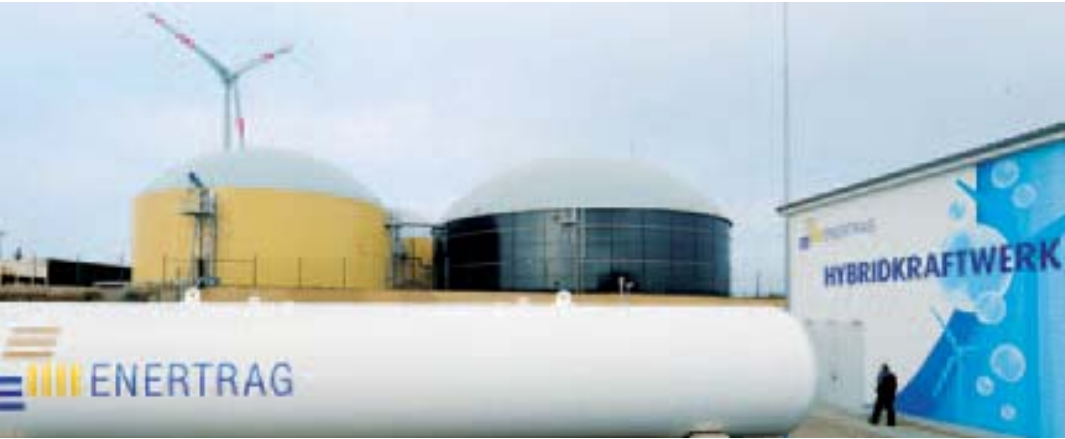
The world's largest hybrid power plant for generating hydrogen from excess wind electricity in Prenzlau near Berlin.
