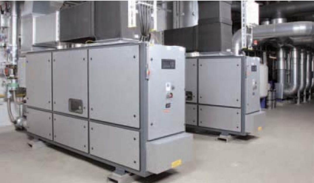
The two ESS combined heating and power units together provide 280 kWel and 414 kWth and achieve efficiencies of more than 90 percent.
