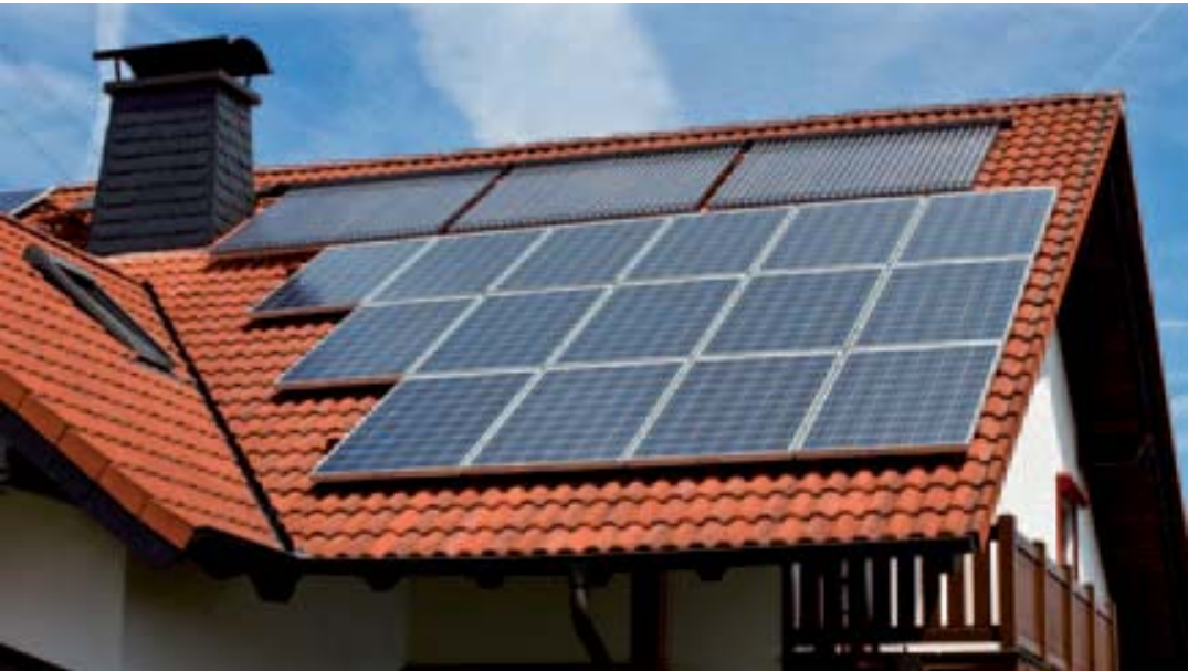
Sustainable revolution on the roof: Solar collectors for DHW and backup heating and photovoltaic modules for generating electricity are a common sight in many places.
