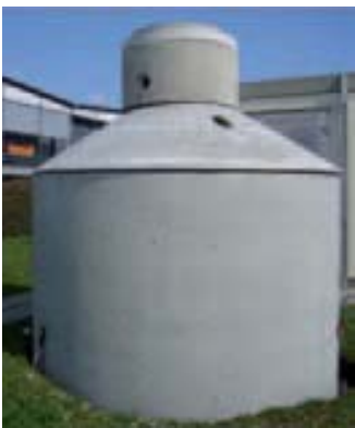
Forming ice in storage tanks of typical size for single-family homes releases as much energy as contained in 120 liters of fuel oil.
